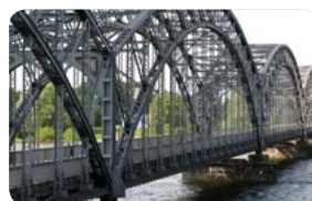
Stahlindustrie | Steel industry
