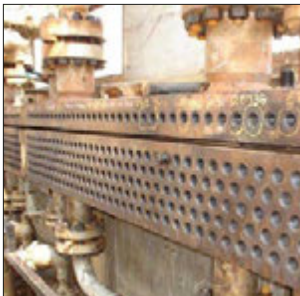
FinFan cooler before maintenance
